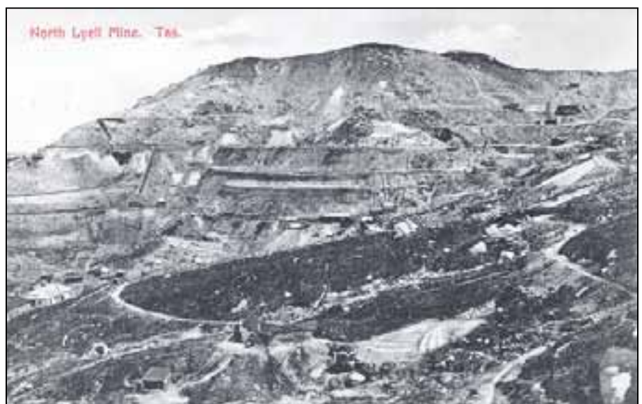
The scene of the disaster, on the eastern side of the ridge which separates Queenstown from Gormanston. Here were both the Mt Lyell mine (the open cut) and the North Lyell mine (an underground mine).
