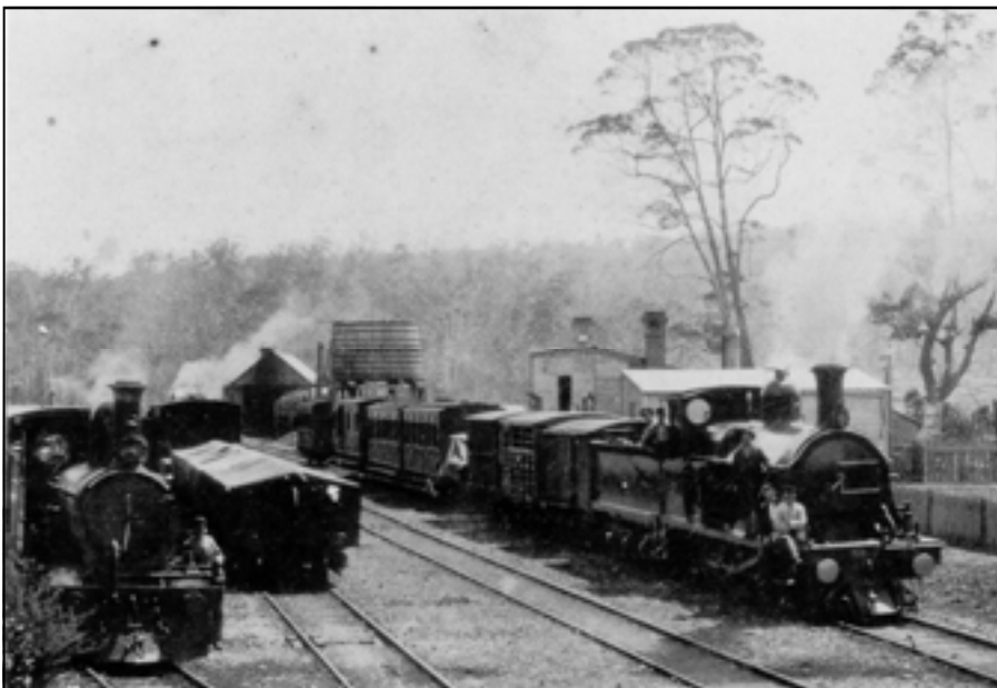
EBR trains at Guildford Junction, where the light rail from Burnie gave way to the new heavier rail on the line to Zeehan and where engines were often changed in consequence.
