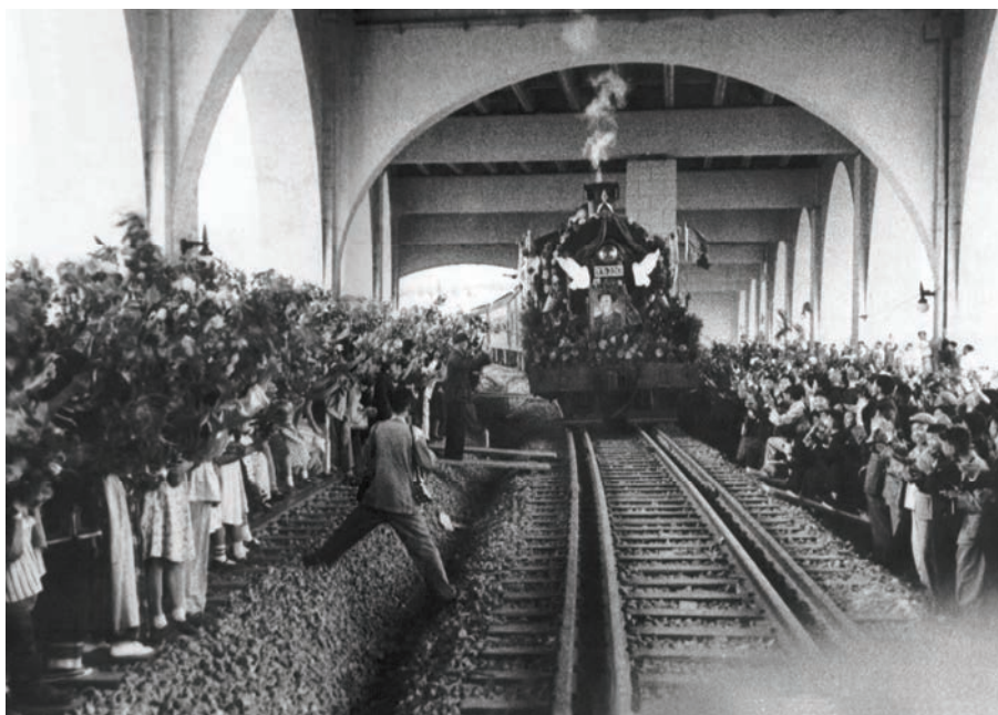
Figure 10. Opening of Wuhan Yangtze River Bridge, 15 October 1957
