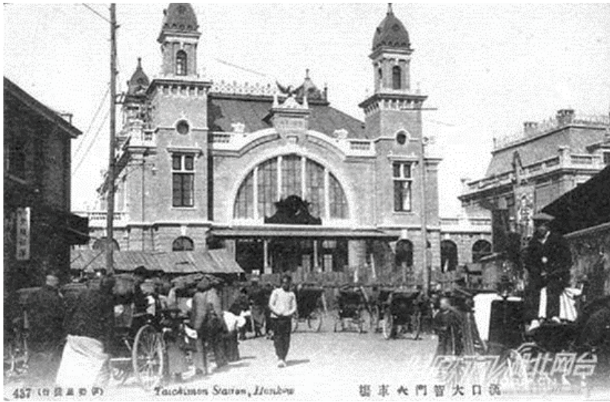
Figure 3 Dazhimen station, Hankou
