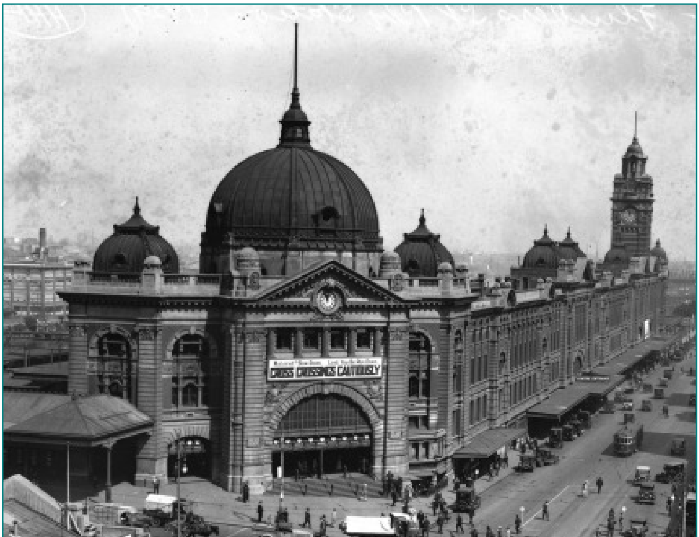
CENTRAL STATION IN MELBOURNE, 1927
