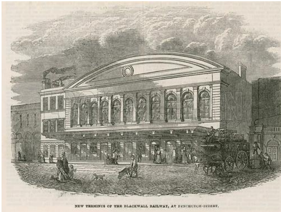
NEW TERMINUS OF THE BLACKWALL RAILWAY, AT FENCHURCH-STREET.
