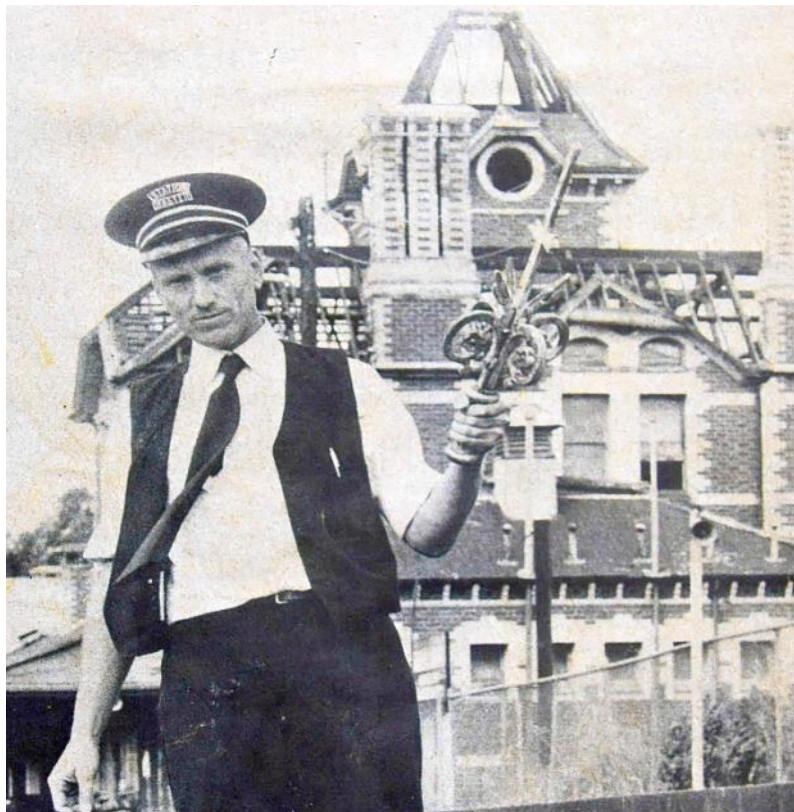
SM George Pryor in front of the partially demolished tea-rooms and tower - Benalla Ensign photo
