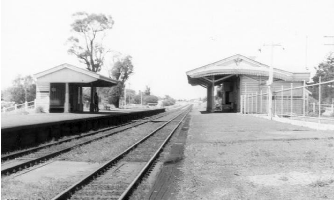
Karrakatta (1897?), looking towards Perth. The cemetery is to the right and defence reserve to the left. Photo courtesy Rail Heritage Western Australia .
