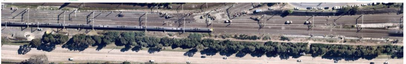
Rookwood station and the cemetery lines, as shown on past maps and present aerial photographs
